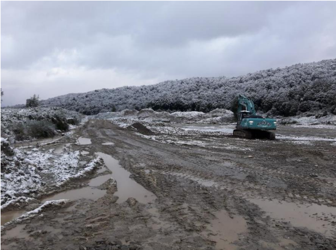
Site earth works underway onsite preparing for surface infrastructure installation
