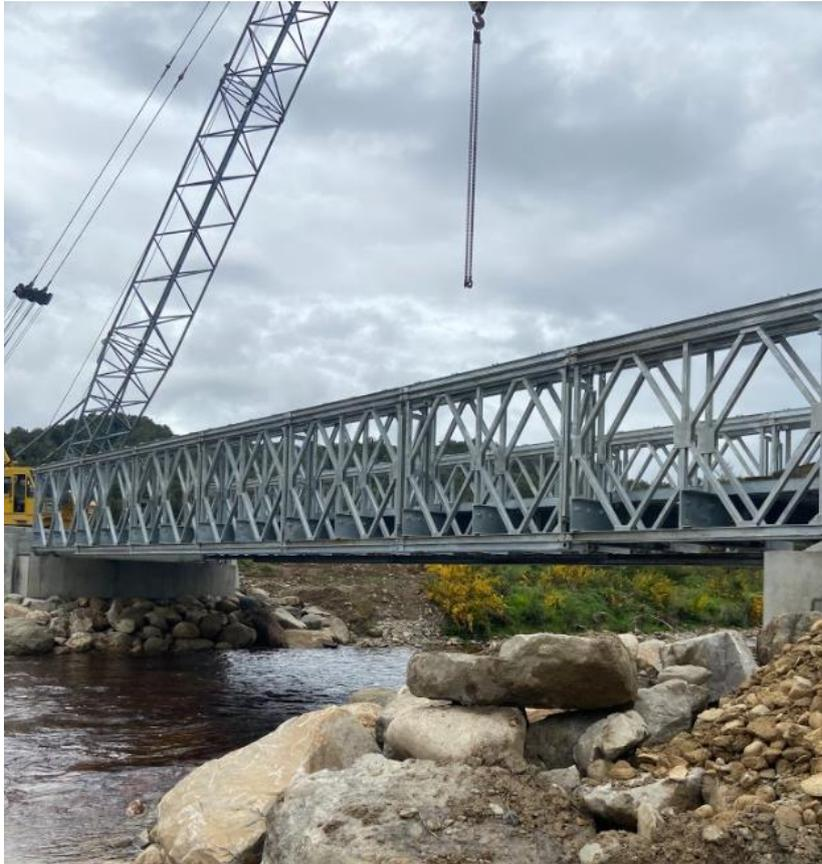
The 21.5 metre Bailey bridge over the Snowy River weighs 36 tonnes and will provide all weather access to the site.
