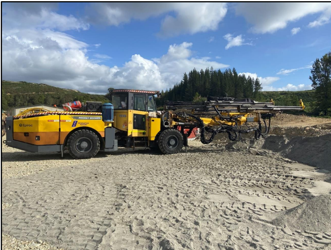
Refurbished Epiroc Jumbo Drill arrived onsite the 27 th of November
