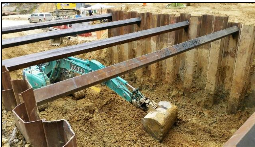
Main Tunnel access 27 th of November
