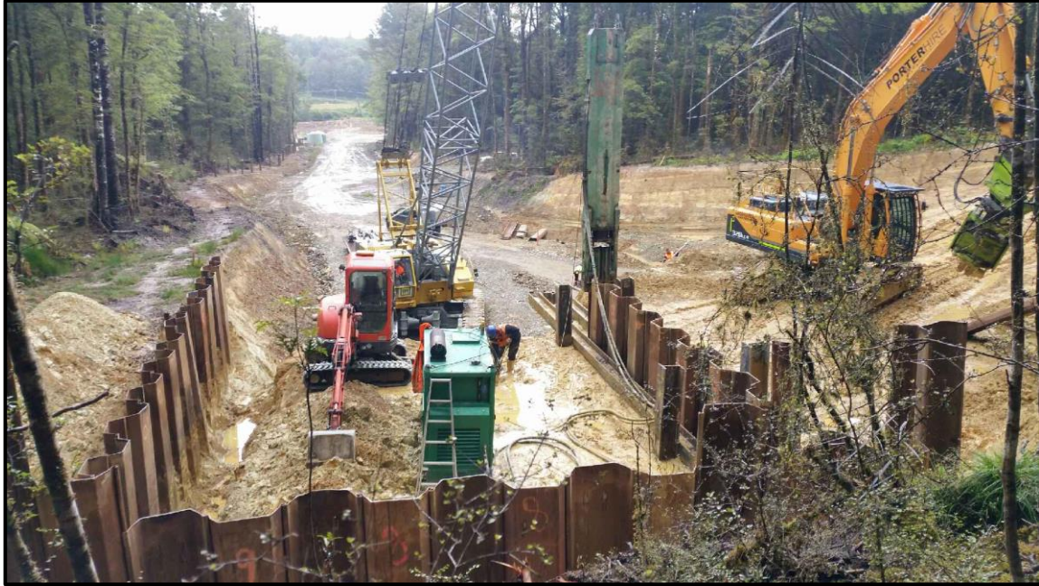
Main Tunnel Sheet piling in progress in mid-November
