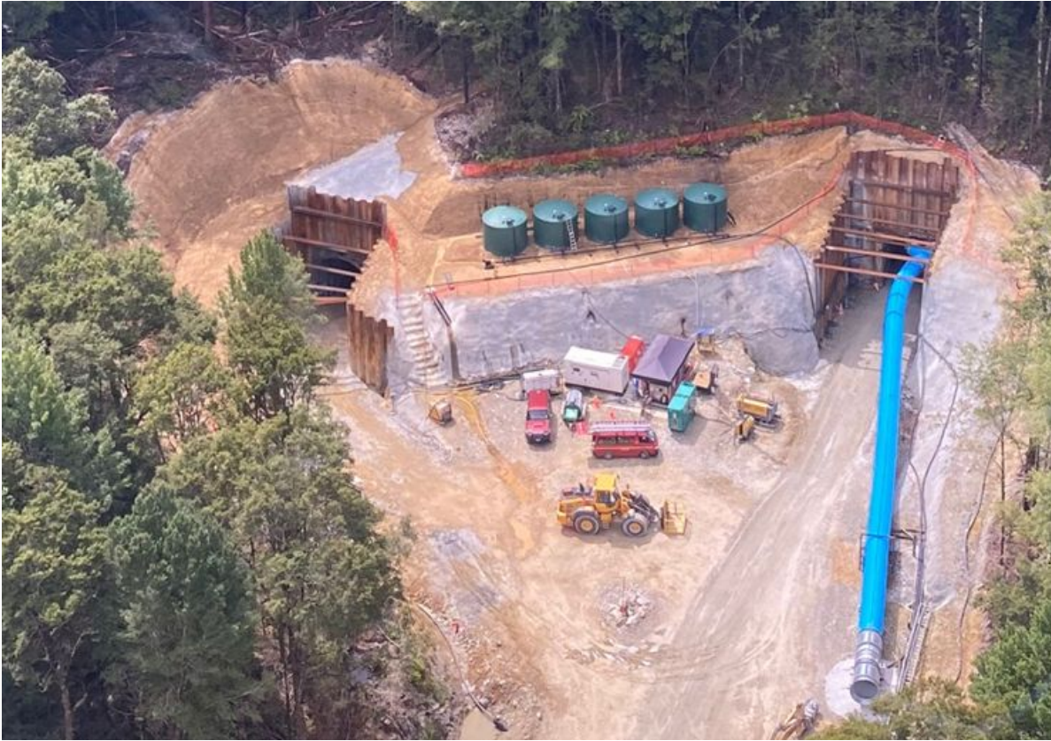
Photo 1 – Aerial photo of North (left) and Main (right) portals.
