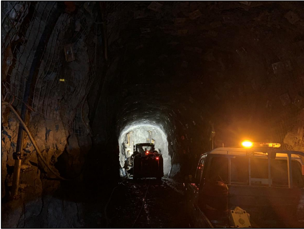
Jumbo Bolting in North Decline
