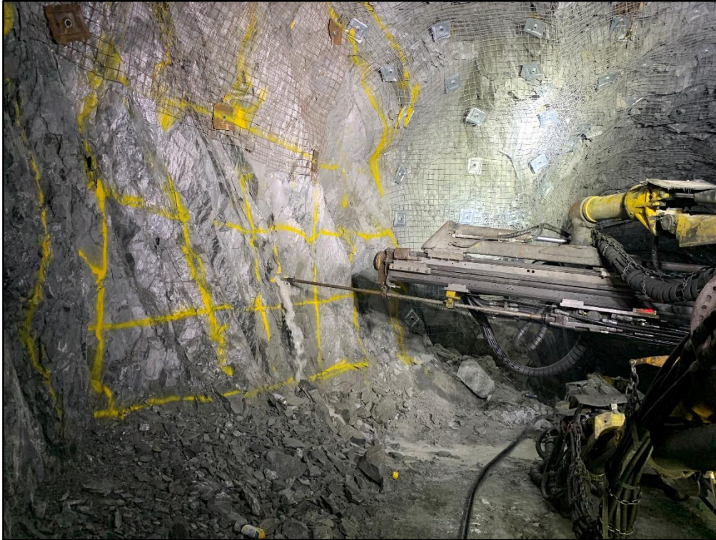
Drilling in Cross-Cut 8
